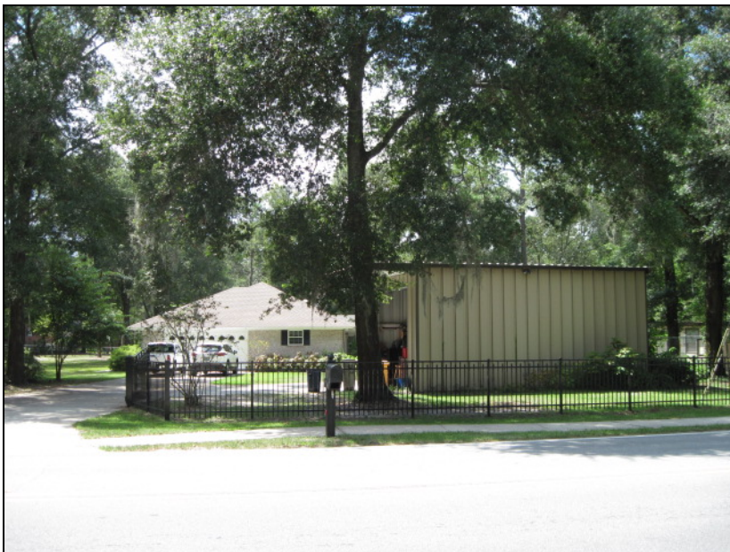
Home located just north of the Julington Creek Road and Aladdin Road intersection.
